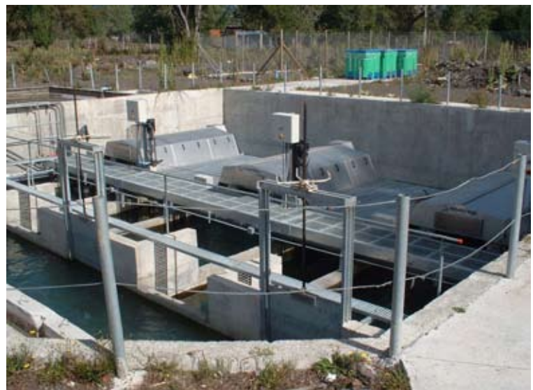
Outlet filtration from salmon farm. 3 pcs HDF2007-2H (without tank)
